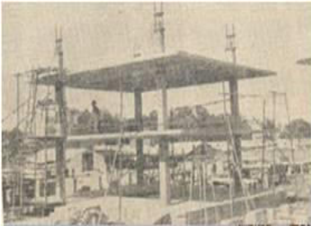
Fig.3: Lift Slab
