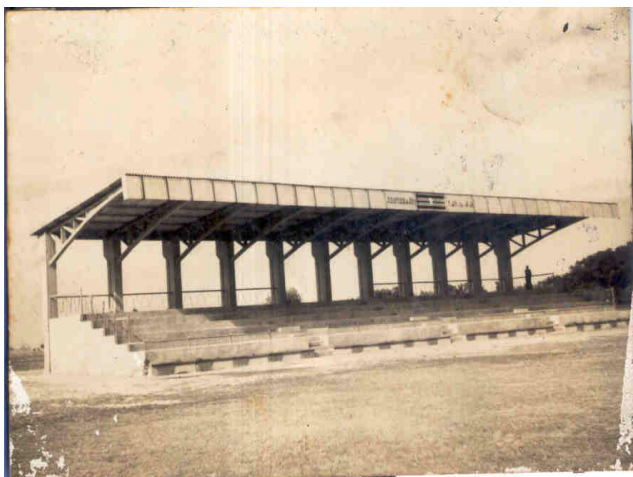
Fig.4: PSC Cantilever Truss
