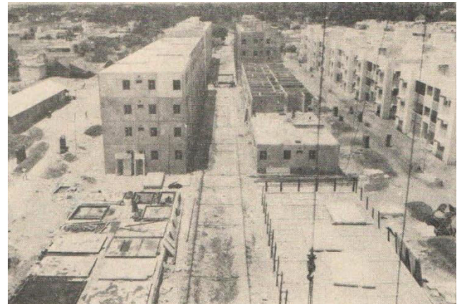
Fig.10: Large Panel Prefab (TNHB Chennai)
