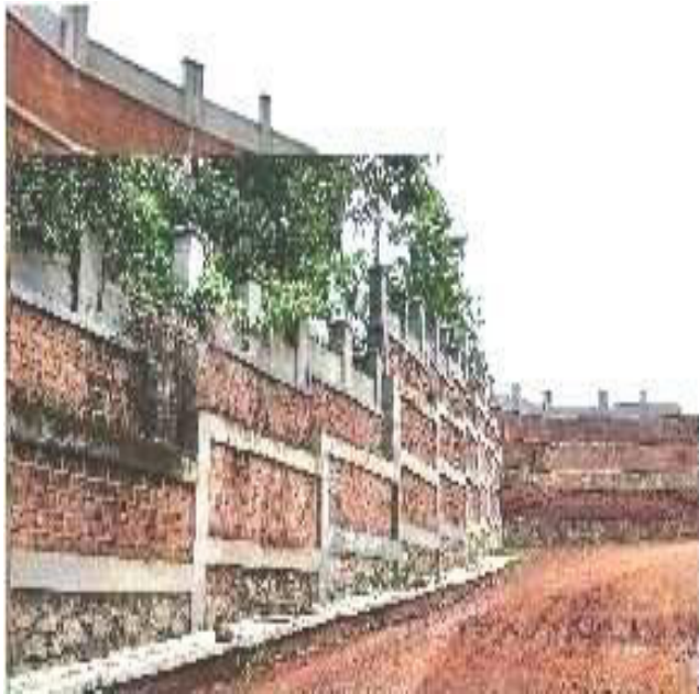
Fig.11: Reinforced Earth Retaining Wall
